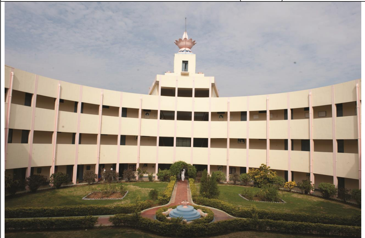
ANANTAPUR CAMPUS MAIN BUILDING (Inside view)
