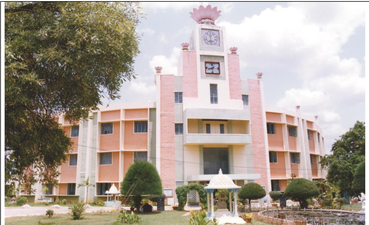
ANANTAPUR CAMPUS MAIN BUILDING (Outer view)
